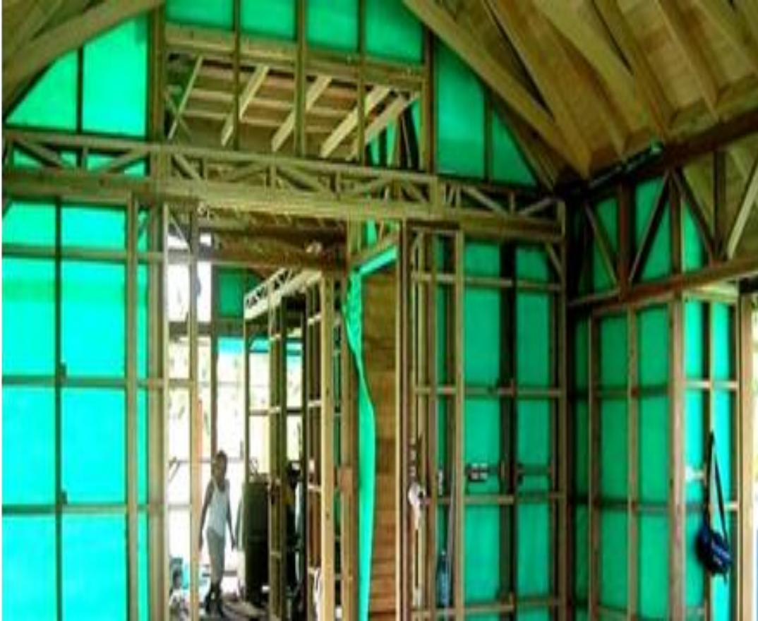
Ready for Thermal Insulation
