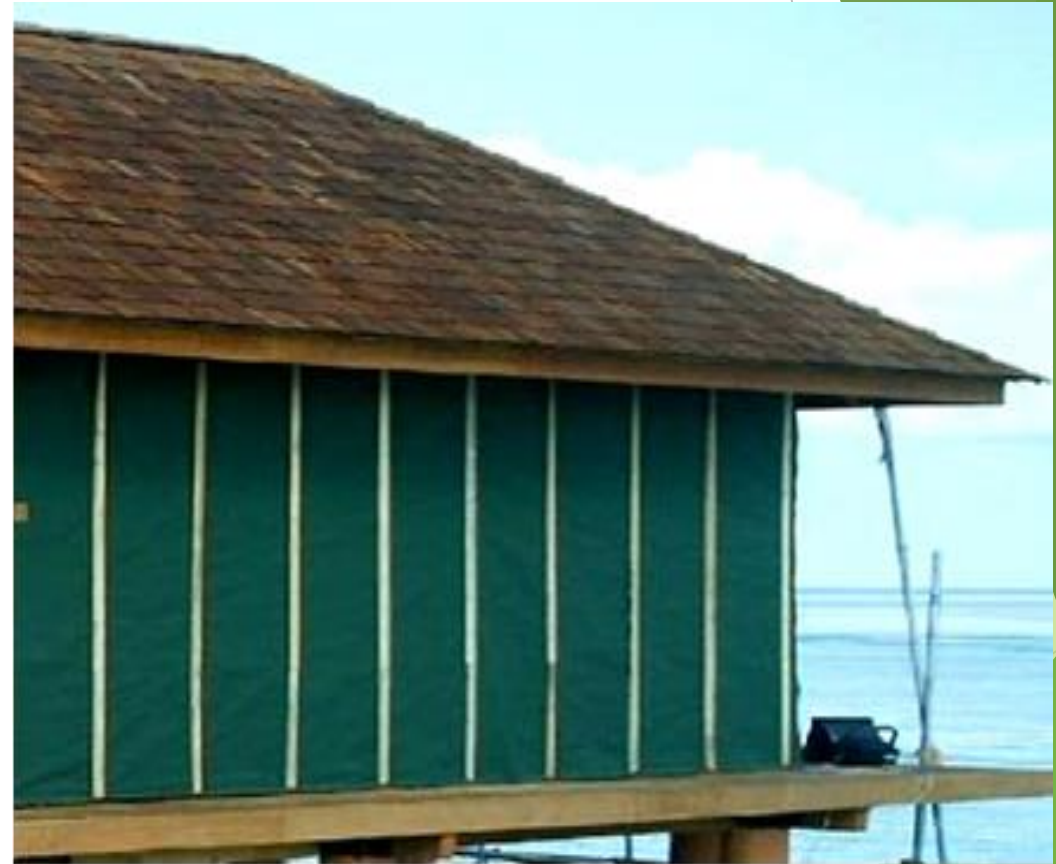
Ready for External Cladding
