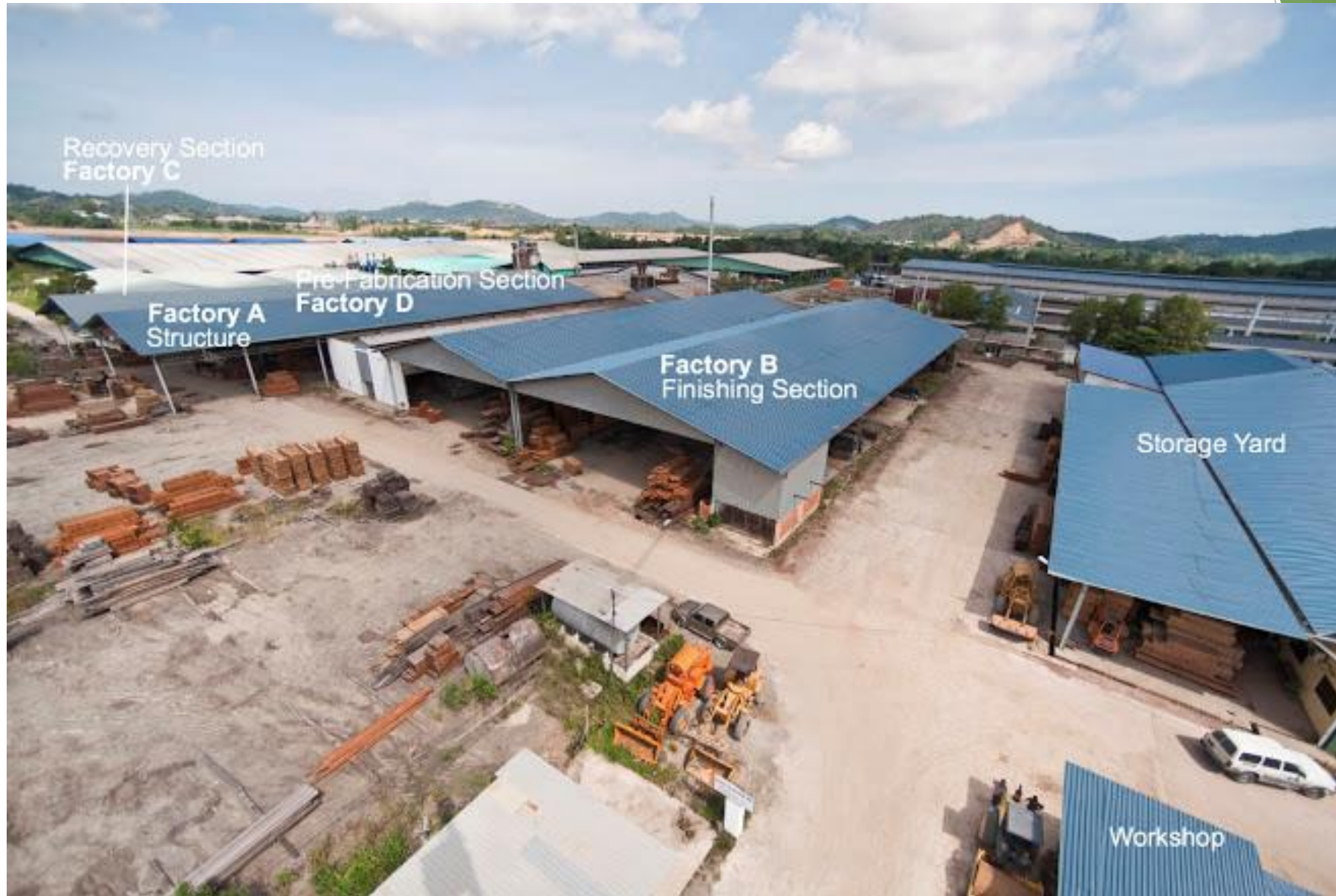
Aerial view of factory in Kota Kinabalu, Sabah
