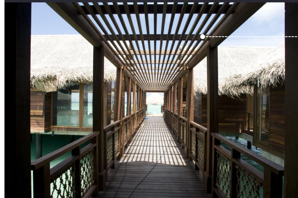
Timber Trellis with Aluminum Rod
