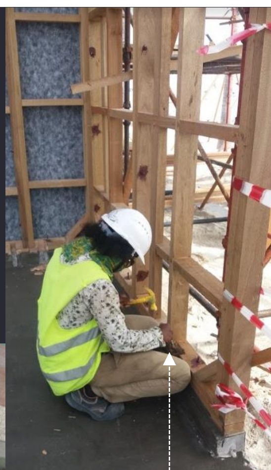
Application of anti-rust substance to all exposed metal bolt and nut
