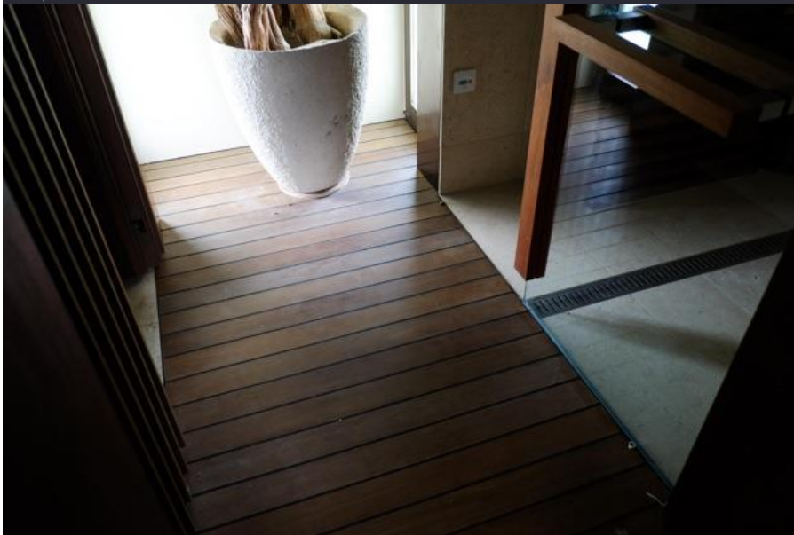
2 Floor board with Polyurethane Sealant
