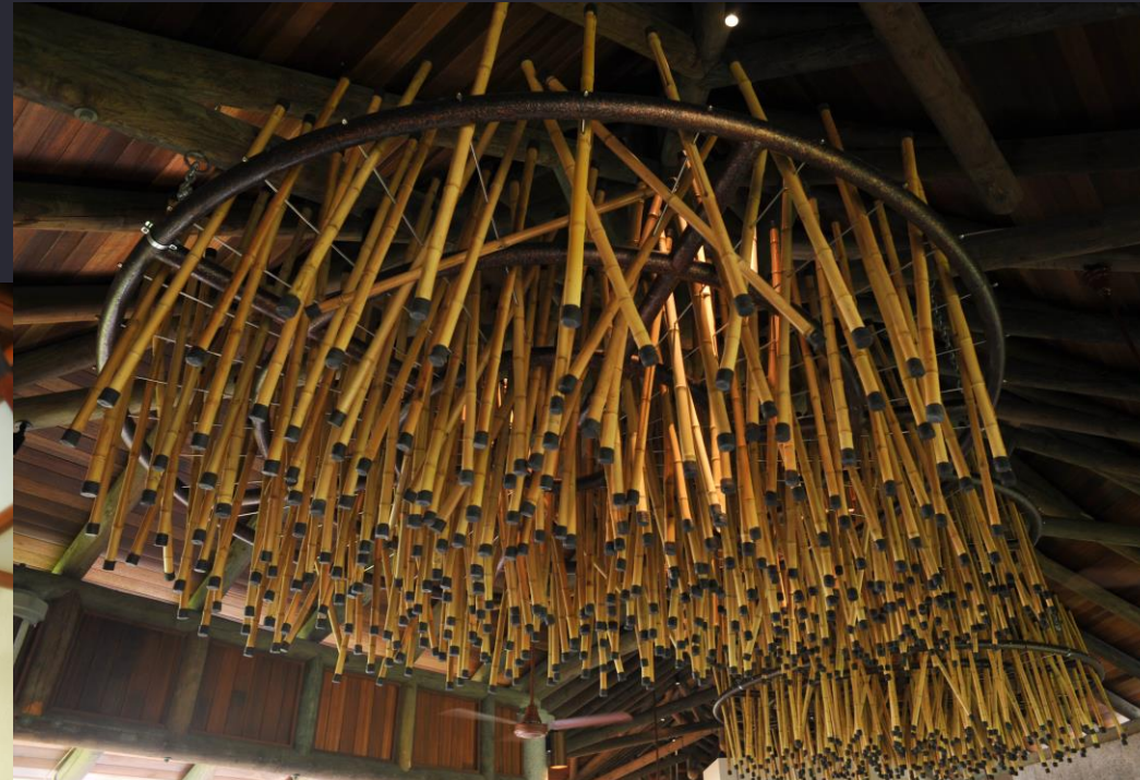
Restaurant Accent Ceiling Feature – Hangings Bamboo Sticks on tubular metal framing
