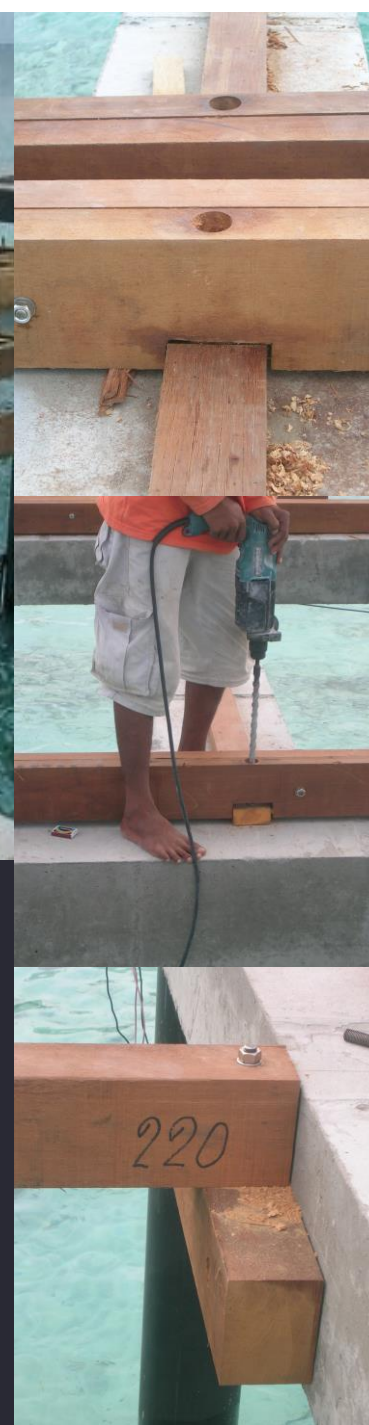
Drilling of timber joist into concrete beam
