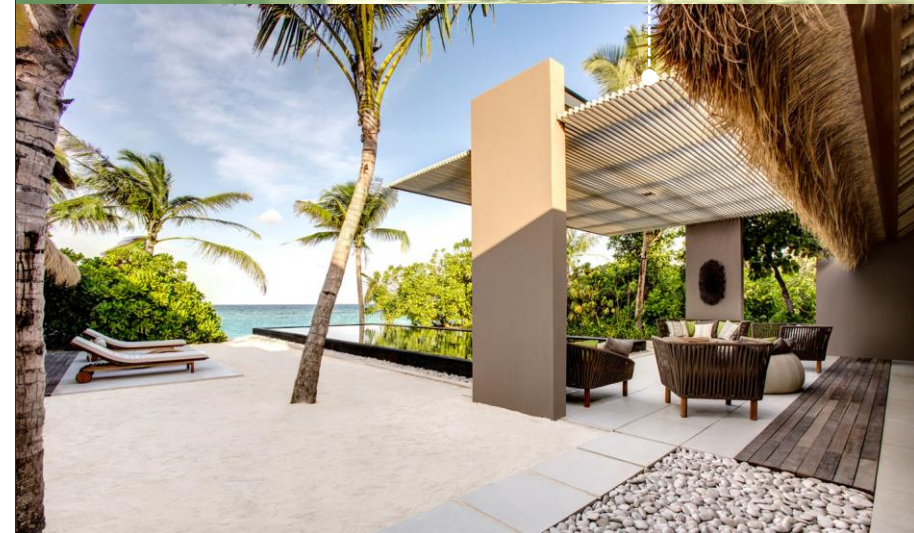
5 Meter span Trellis with Metal I-Beam
