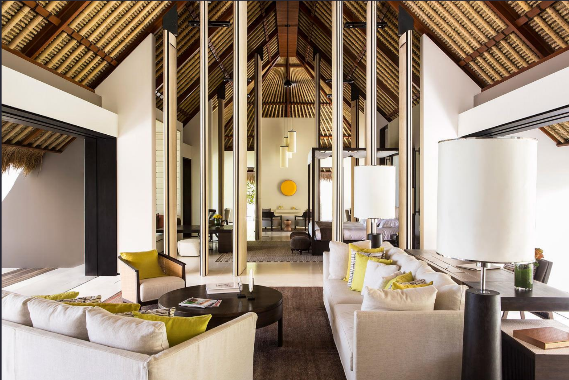
Exposed Cadjan Ceiling Finish with Bamboo Rafter
