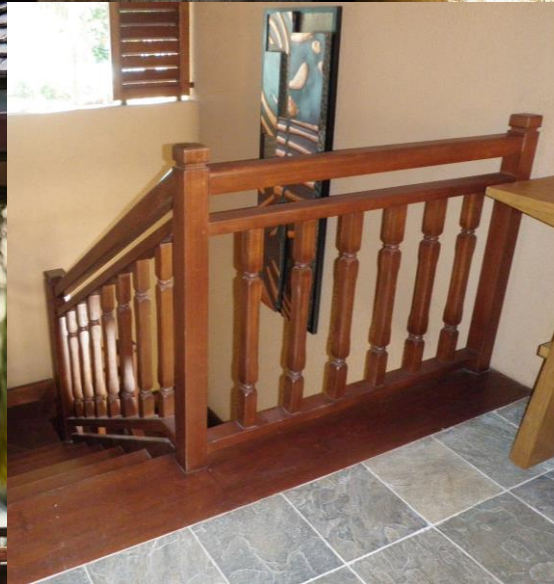
Timber Railing with Profiled Vertical Timber Balustrade Photos from Constance Ephelia Resort - Seychelles
